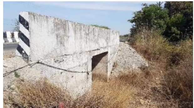
Km. 5+840 of Neemuch-Nayagaon
