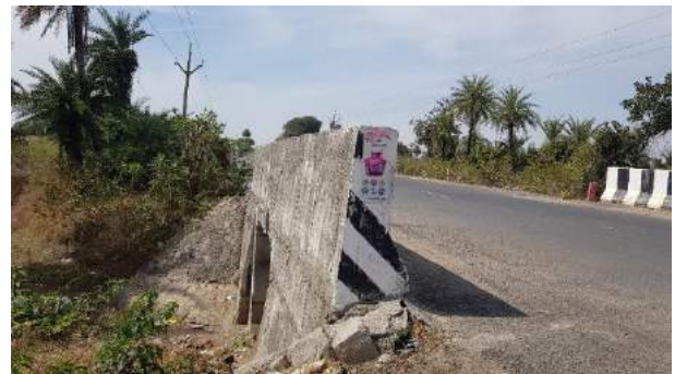
Km. 13+960 of Neemuch-Nayagaon
