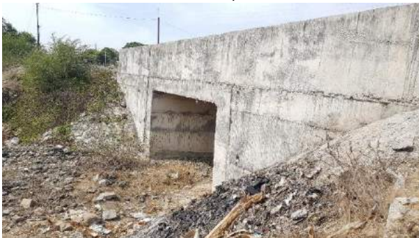
Km. 12+365 of Neemuch-Nayagaon
